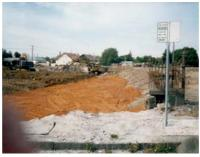
Backfilling operations showing the orange marker layer above the contaminated soil capsule.
