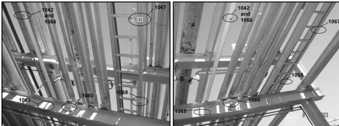
**Figure 3:** 'Hard Points' Used for Photogrammetry
