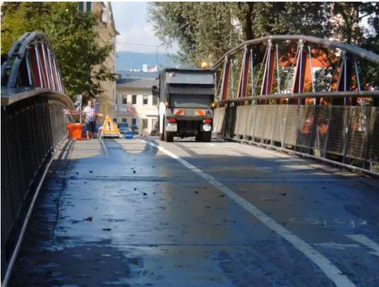
Fig. 11 Excitation of the bridge by a vehicle
