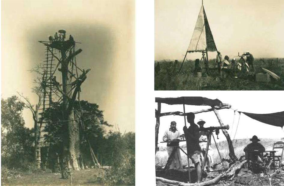
Fig.8 – Cartographic station, Boabá, 16 m (left); Plane table and alidad (up); Drawing the cartographic document (down)
