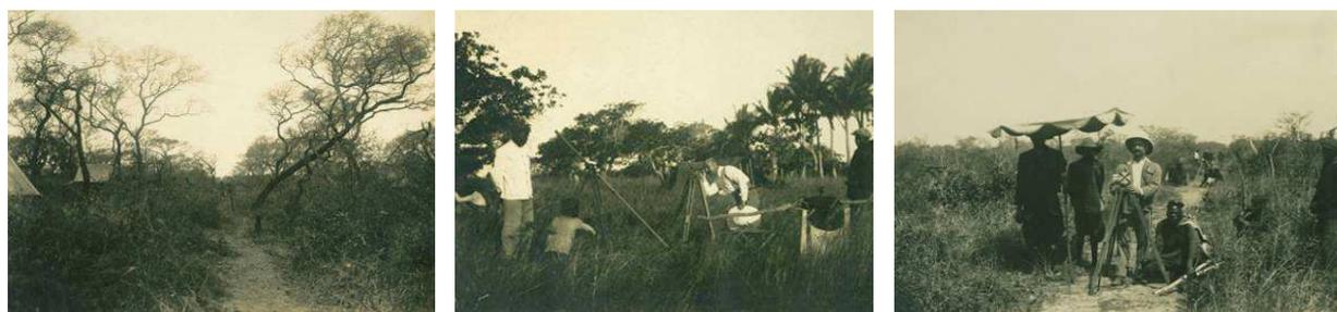
Fig.7a – some procedures of measuring baselines: (from left to right) to make way to measure Manhiça baseline; leveling; alignment of the tripods
