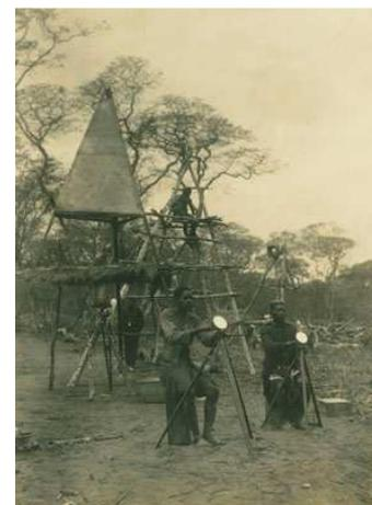
Fig.6a – part of the triangulation chain, N Tungluane tower and projectors, Landins pointing heliotropes
