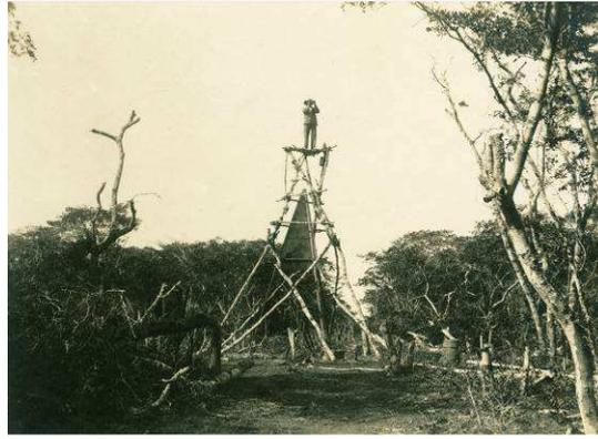
Fig.6 – Checking inter-visibility from the top of a tree. Measuring with the sextant (from left to right)
