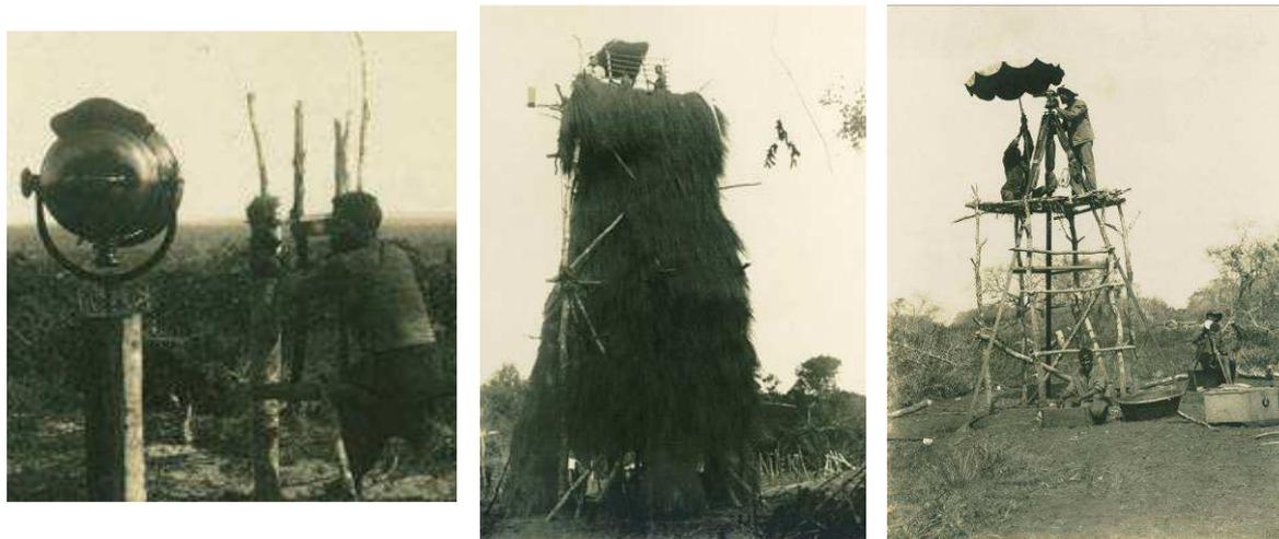
Fig.6b – projector; 10 m tower lined with straw; measuring angles (up, down, from left to right)
