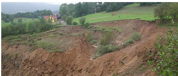
Landslide in Tenczyn
