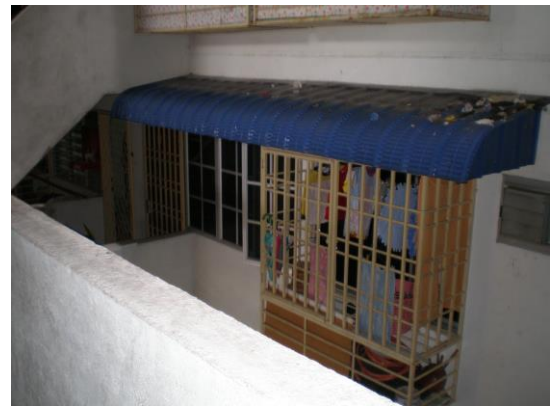
Fig 16 Cage laundry along open air well
