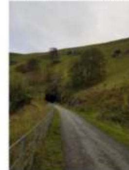
Figure 4.11: Crossbrook tunnel approach
