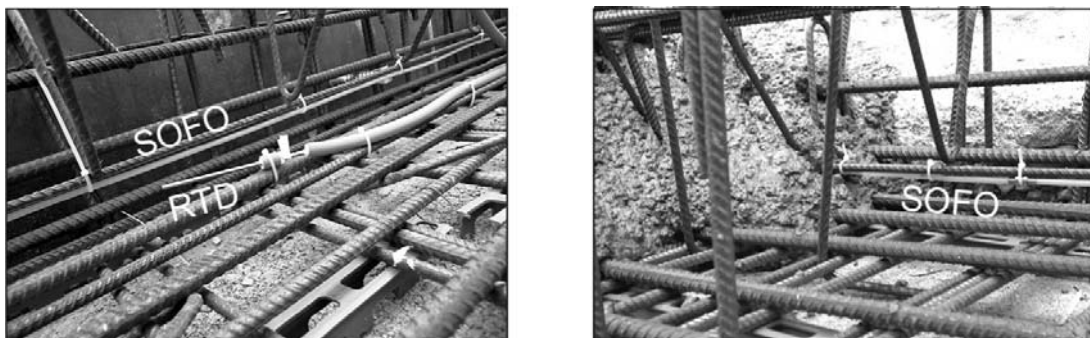
Fig. 6: Installation of the sensors and pouring of the concrete
