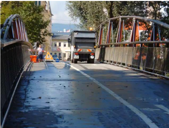
Fig. 11 Excitation of the bridge by a vehicle
